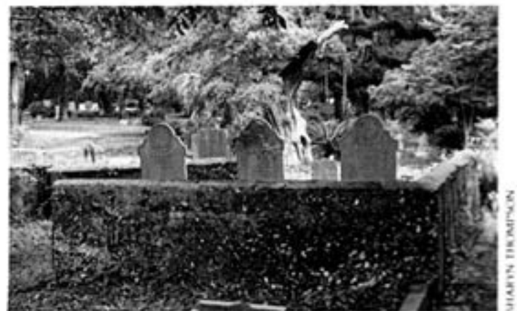
This tabby wall is significant to the historical character of the cemetery.
