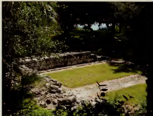
1750s stone foundations of Fort San Marcos de Apalache
