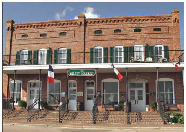
The Grady Building, Water Street, Apalachicola. (Image courtesy of the Apalachicola Chamber of Commerce)
