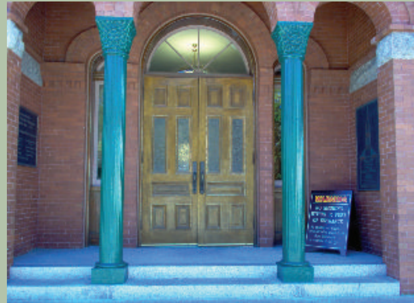
To protect it from storm damage, the historic Nassau County Courthouse was the subject of a Hazard Mitigation Grant application for window protection. NASSAU COUNTY
