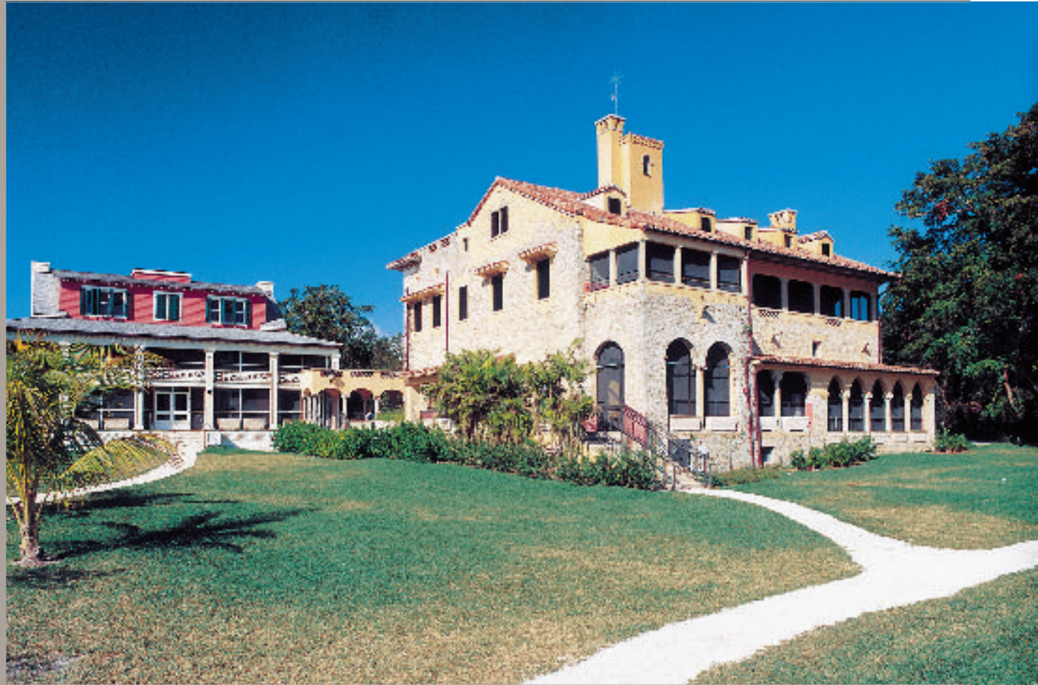
Miami's Deering Estate (shown above and on opposite page) was restored after sustaining major damage during Hurricane Andrew.
