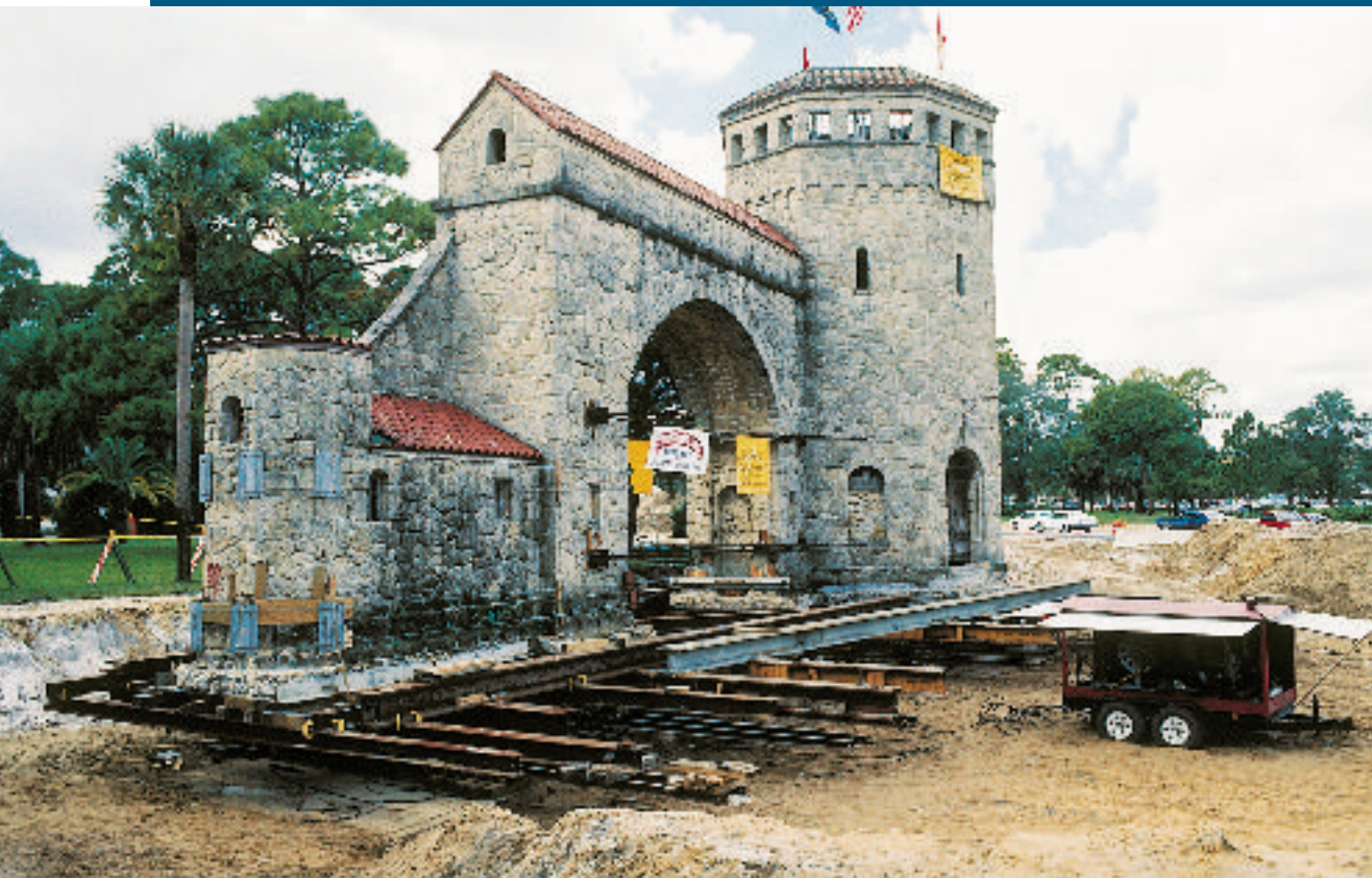
The Terragonna Arch in Daytona Beach was relocated as mitigation for widening of a U.S. highway.
